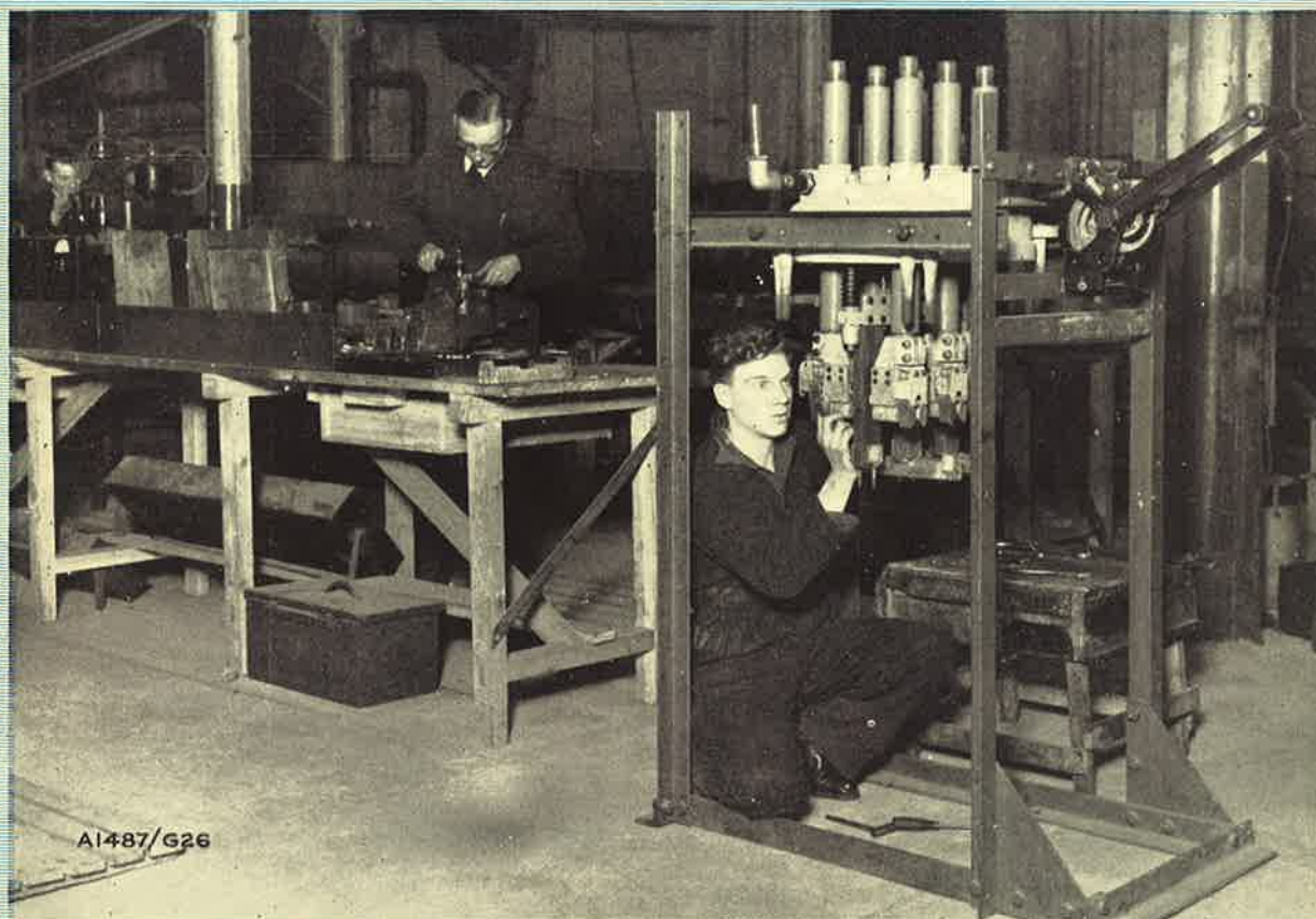
(Below) Fitting and assembly of a 1,200 ampere 11,000 volt Oil Circuit Breaker.
